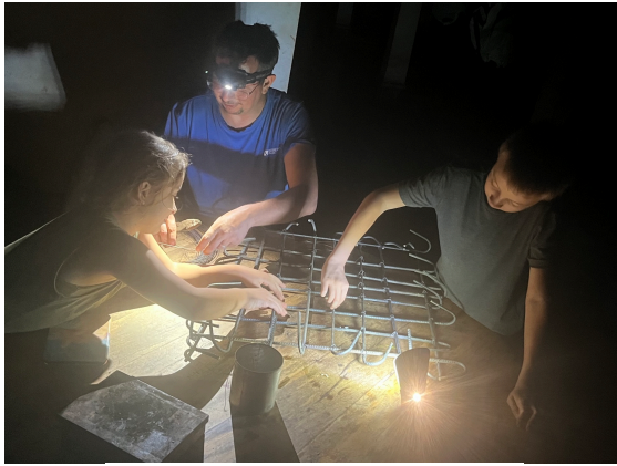
Tying rebar by solar light
